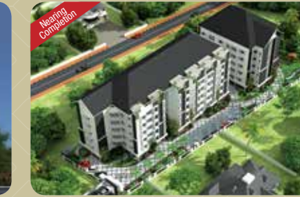
HIGHWAY AVENUES NH 47 Bypass - Kochi
